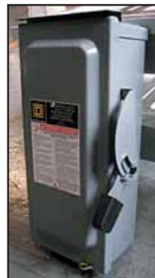
It is strongly recommended that all 220 and 440VAC connections be connected through a power disconnect switch (example seen at left) for use with either CNC Router spindle and/or vacuum pump setup. This switch is required for safety and to meet National Electrical Codes. A licensed electrician should perform this installation.
